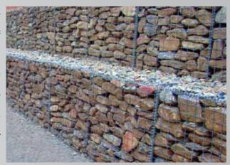
(Note: Retaining walls are permanent structures typically constructed at a toe of slope or to retain backfill.)
